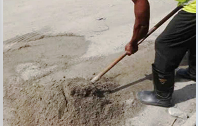
Man patching road...Nkayi locals say menial jobs are not a reliable source of income. Image by Bassey
