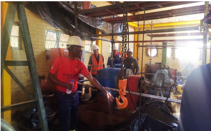
Workers repair a pump at Umzingwane, upgrading Bulawayo’s aging water system. | Photo: Sharon Sibindi/ The Citizen Bulletin
